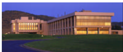
Zentrale in Denver/Colorado, USA
